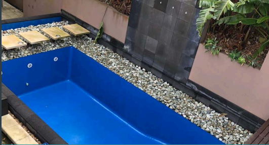
POOL REPAINTED IN EPOXY POOL PAINT - DEVONPORT COLOUR
