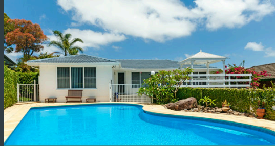
POOL REPAIRED, SEALED & REPAINTED IN EPOXY POOL PAINT - PACIFIC BLUE COLOUR
